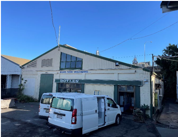
Photo 4: Overview Doyles Warehouse
