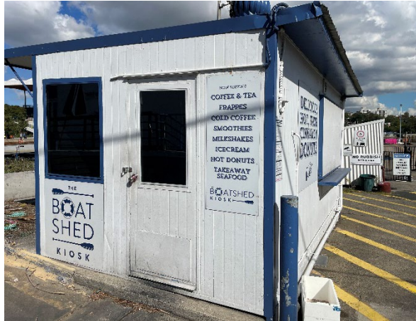
Photo 134: Overview of Kiosk building – 30/04/26
