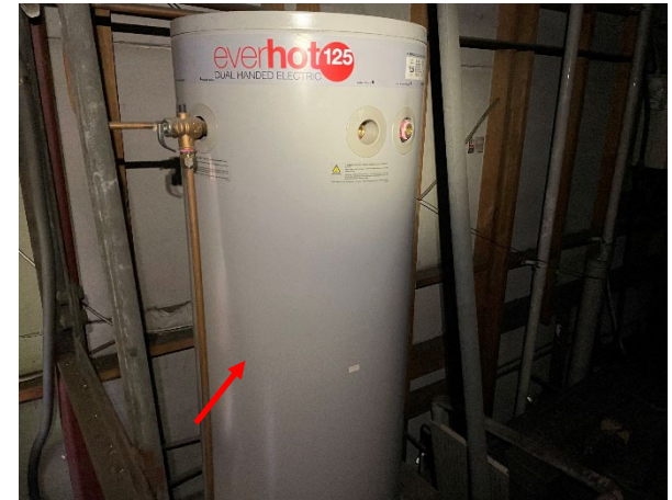
Photo 24: Internal, Doyle's Warehouse ceiling cavity, hot water heater – assumed SMF insulation core
