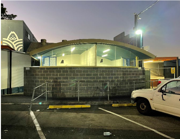
Photo 40: Overview of Public Toilet
