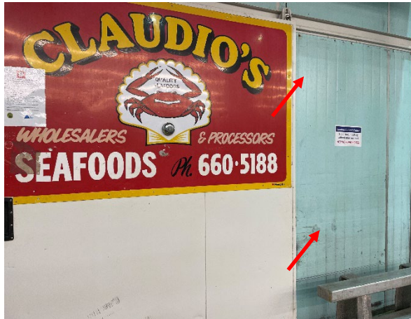
Photo 83: Internal, ground level Claudio's cool room, walls – assumed SMF insulation
