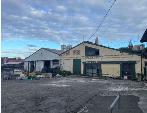
Photo 103: Overview of Building A – 01/05/26
