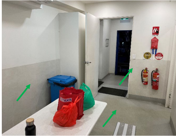
Photo 92: Internal, level 1 lunchroom, walls and floor – non-asbestos containing vinyl sheet
