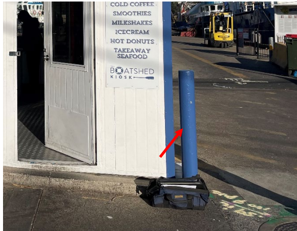
Photo 95: External, traffic bollards – lead based blue paint with yellow undercoat
