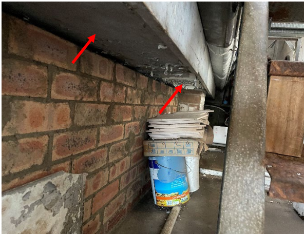
Photo 88: Internal, level 1 storeroom, original eaves (partially removed) – asbestos containing fibre cement sheeting
