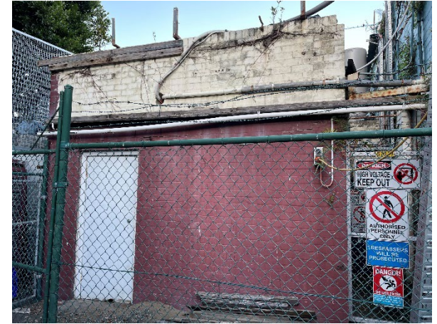
Photo 45: Inaccessible secondary main switch room and electrical substation
