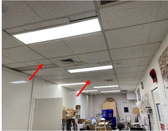
Photo 80: Internal, level 1 ceiling – assumed SMF ceiling tiles
