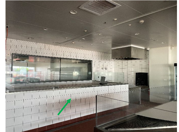
Photo 111: Vic's Meats, internal, ground floor, butchers' area, behind white tiled walls – non-asbestos containing fibre cement sheeting
