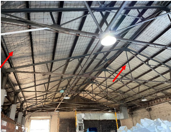
Photo 22: Internal, Box Recycling Warehouse, underside of roof – assumed SMF sarking
