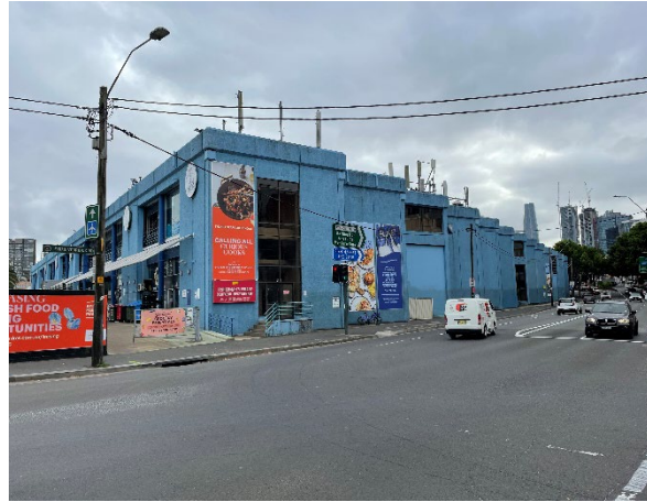
Photo 62: Overview of Building D looking north
