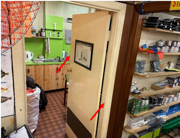
Photo 34: Internal, Net & Tackle, door frame – lead based cream paint
