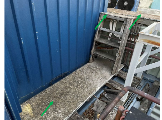
Photo 93: External, level 1 roof access, steps and walkway – non-asbestos containing compressed fibre cement
