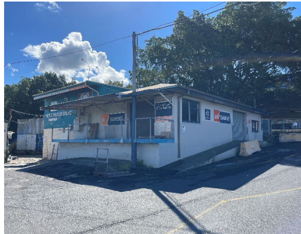
Photo 113: Overview of Building B – 30/04/26
