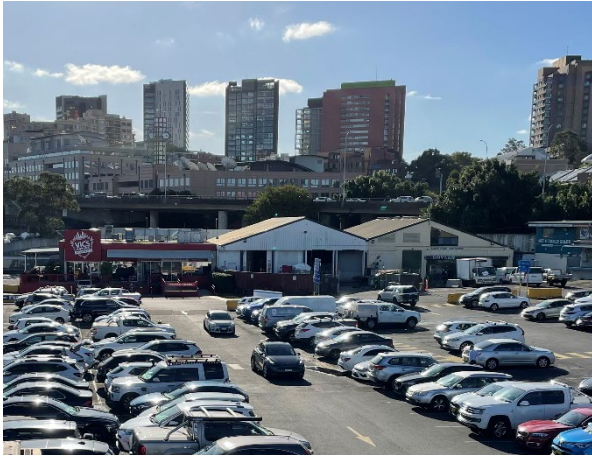
Photo 1: Overview Building A
