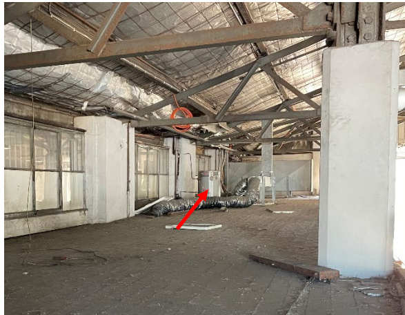
Photo 23: Internal, Box Recycling Warehouse roof to office area, hot water heater – assumed SMF insulation core
