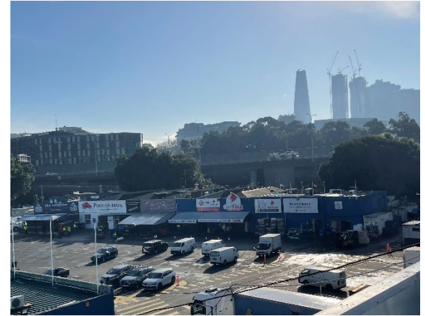
Photo 39: Overview Building C
