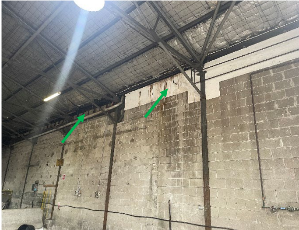
Photo 109: Internal, between Box Recycling Warehouse and Doyles Warehouse – infill panel to the Besser block wall and gutter – non-asbestos containing cement
