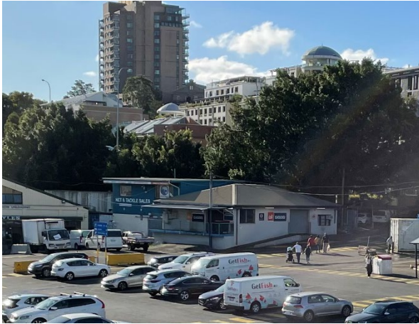
Photo 25: Overview of Building B
