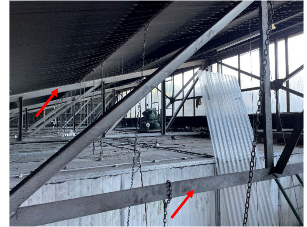
Photo 57: Internal, Poulos Bros ceiling cavity, metal framework to saw tooth roof – lead based grey paint
