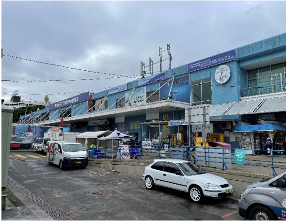
Photo 61: Overview of Building D looking south
