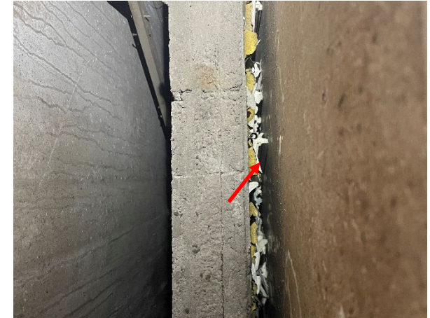
Photo 123: Poulos Bros, internal, ceiling cavity, original brick walls – lead based cream paint
