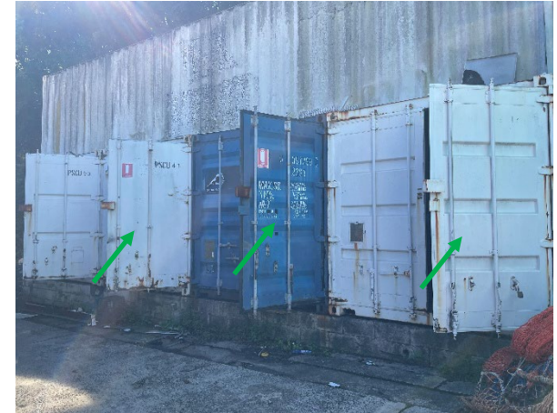
Photo 135: External, northern portion of site, adjacent All Seas, two white and one blue shipping containers – non-lead based white and blue paints
