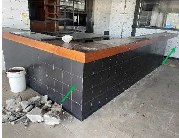
Photo 110: Vic's Meats, internal, ground floor, bar area, behind black and white tiled walls – non-asbestos containing fibre cement sheeting
