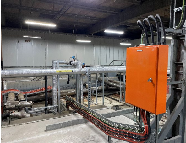
Photo 79: Internal, throughout plant rooms and ceiling cavities, pipework – assumed SMF insulation
